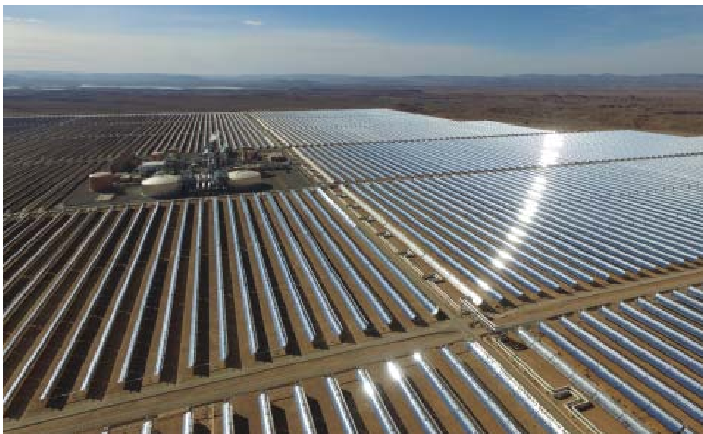
ACWA Power is responsible for the construction and operation of 170 MW of plants as part of the Noor project in Morocco, which generates power using both PV and CSP technologies.
