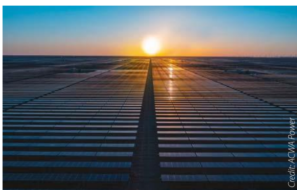
The Sakaka Power Plant in Saudi Arabia, developed by ACWA Power.
